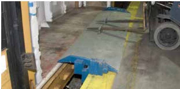
RAIL BOARD PLACEMENT
